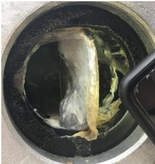
Contaminated pipe (binder) before procedure
