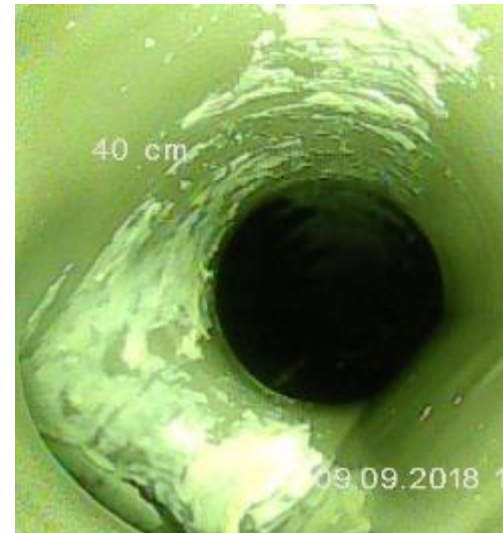
Contaminated pipe after cleaning with system cleaner solution (Vinkoclean SR1)
